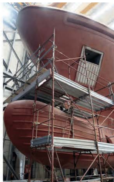
▲ Ice-busting steel is the material of choice for explorer yachts, such as this 500 EXP taking shape in Viareggio
